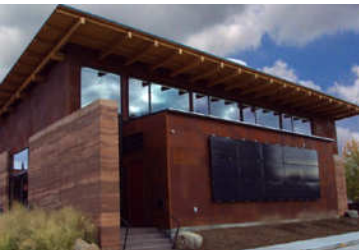
The library's photovoltaic panels are located on the Charles Street rammed earth walls of the new addition.
